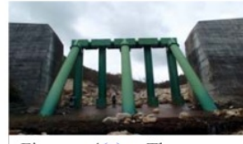
Figure 4(a). The open check dam in the Hachimandani River.
